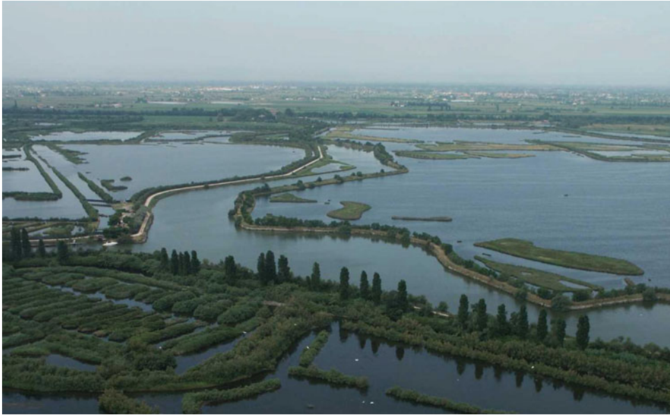
Fig. 15.8 Fish farms in the southern basin of the lagoon (Valle Averte). In the foreground is the system of pools for fish recovery, and in the background is the network of embankments ( photo A. Bondesan)
