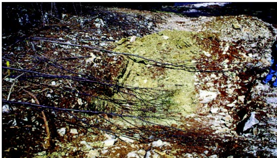
Ph. 3: On the inclined karst plain south of Divača the cave which is also inclined was uncovered during the motorway construction. Both are affected by younger tectonical movement.
