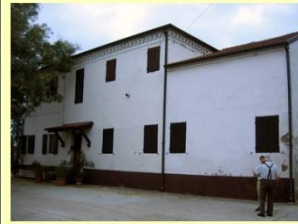
Hydraulic storehouse on the left bank (XVI century)
