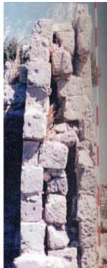
double leaf with transversal connection
