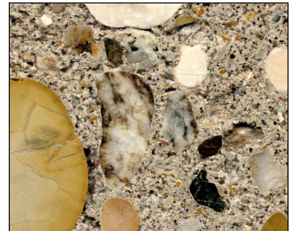
Padova castle concrete beam: entrapped air voids
