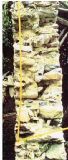
double leaf with transversal connection
