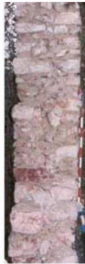
double leaf with transversal connection
