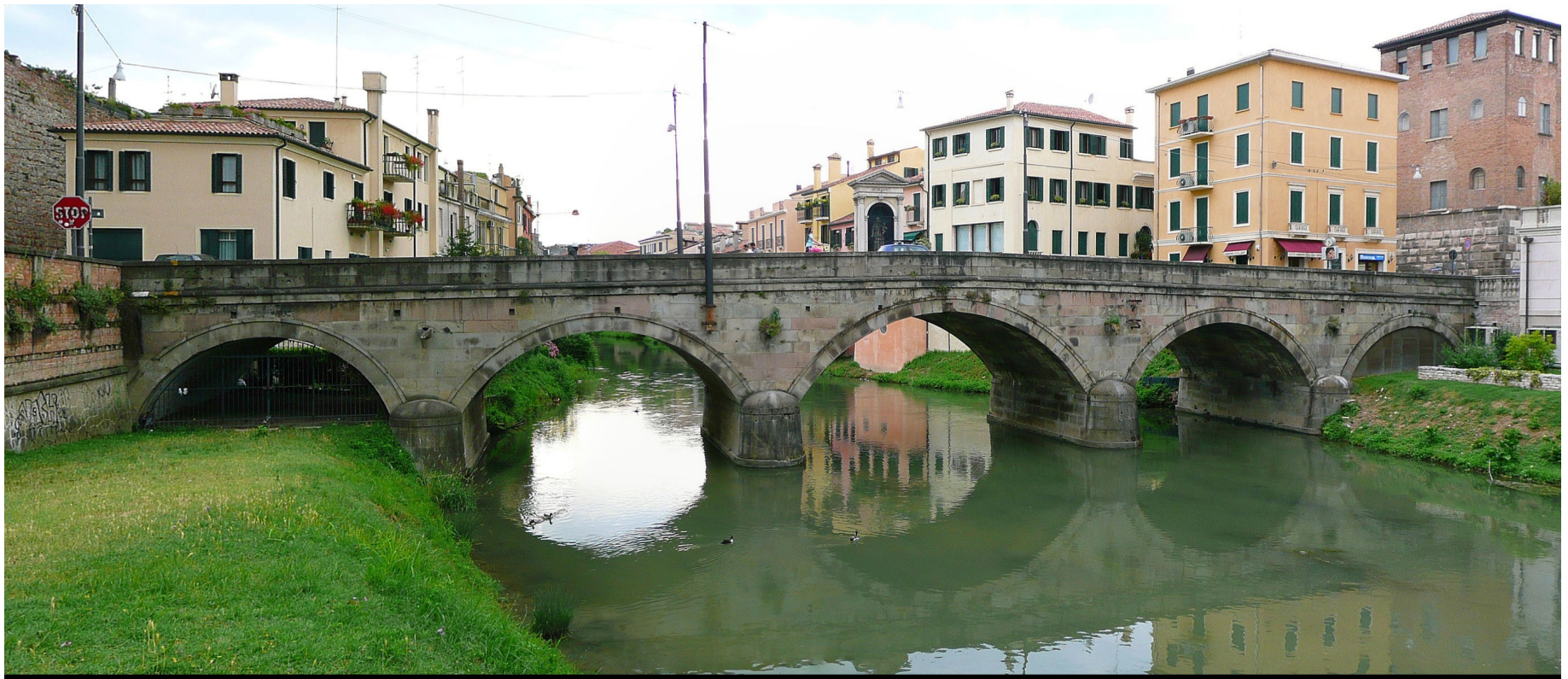
Padua, Molino bridge
