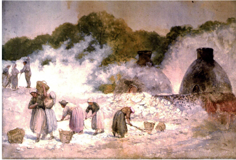
FIG. 1.9 Joseph Aspdin's first cement works at Kirkgate, Wakefield.
