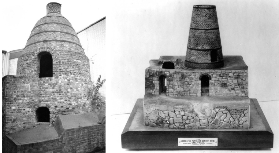
FIG. 1.11 Preserved beehive kiln at William Aspdin's works in Northfleet, Kent along with the photograph of a model of an adjacent kiln now demolished.
