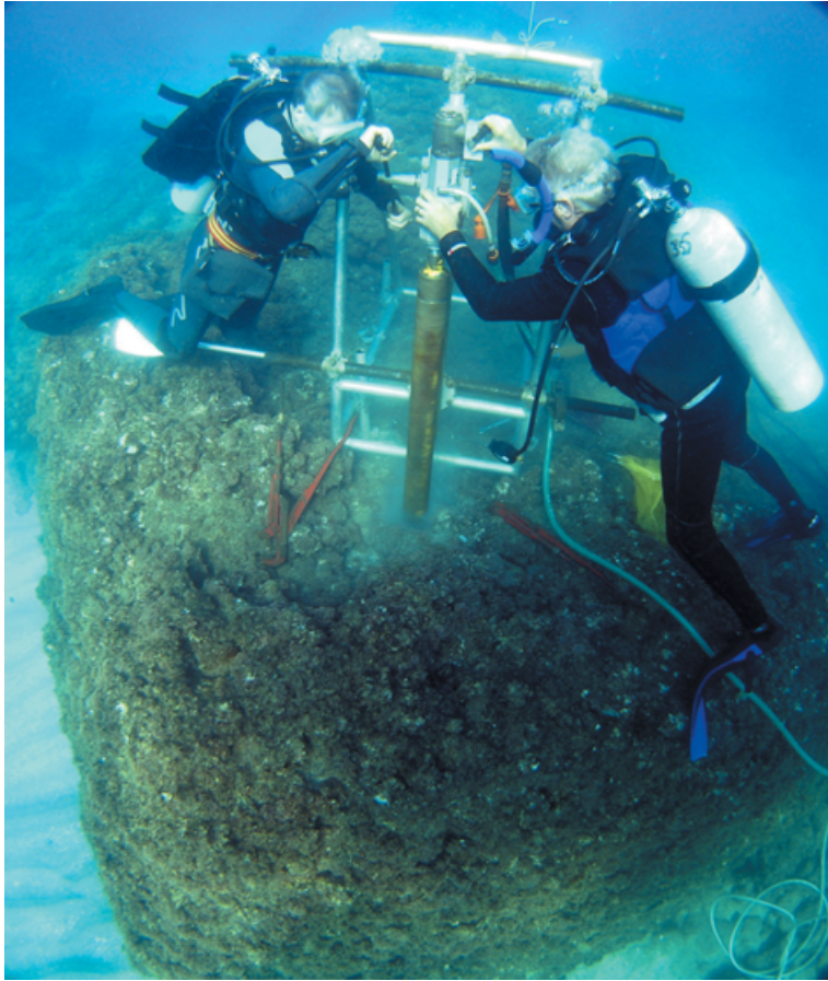
Figure 2. Coring equipment in operation. (G. Votruba)
