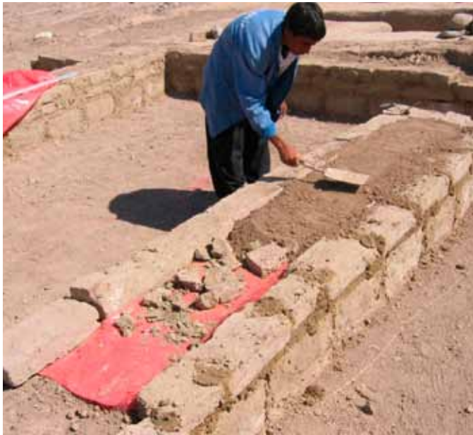
FIGURE 6 The conservation method of treating the walls within the trenches. Photo: Manijeh Hadian, RCCCC
