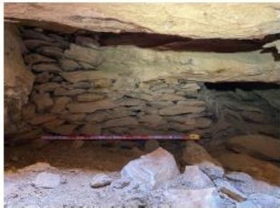
Figure 24—Shoring works inside the mine [SKP-US2] (source: authors).
